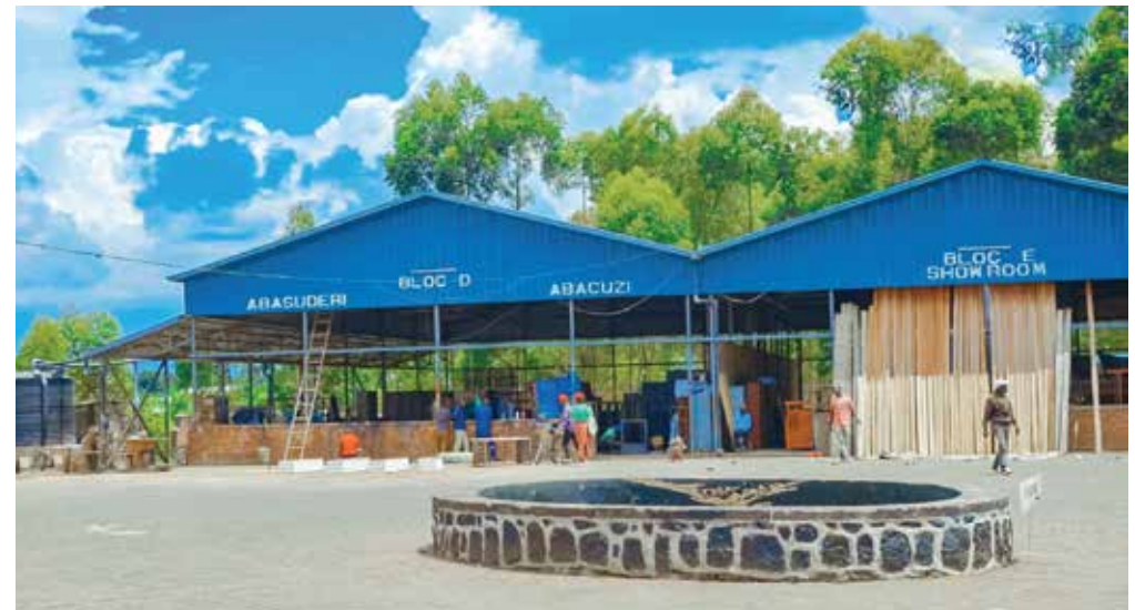
The newly constructed handcraft centre in Musanze town created off-farm jobs for many people.
